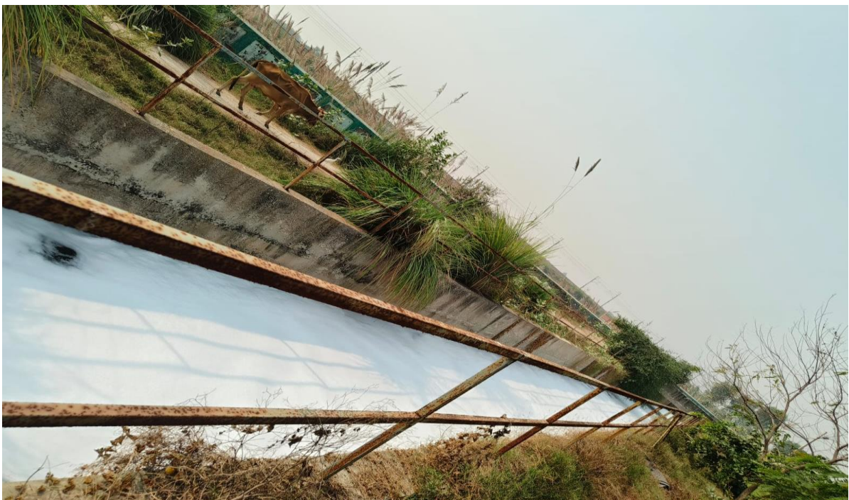
Image 7: STP outlet laden with foam
