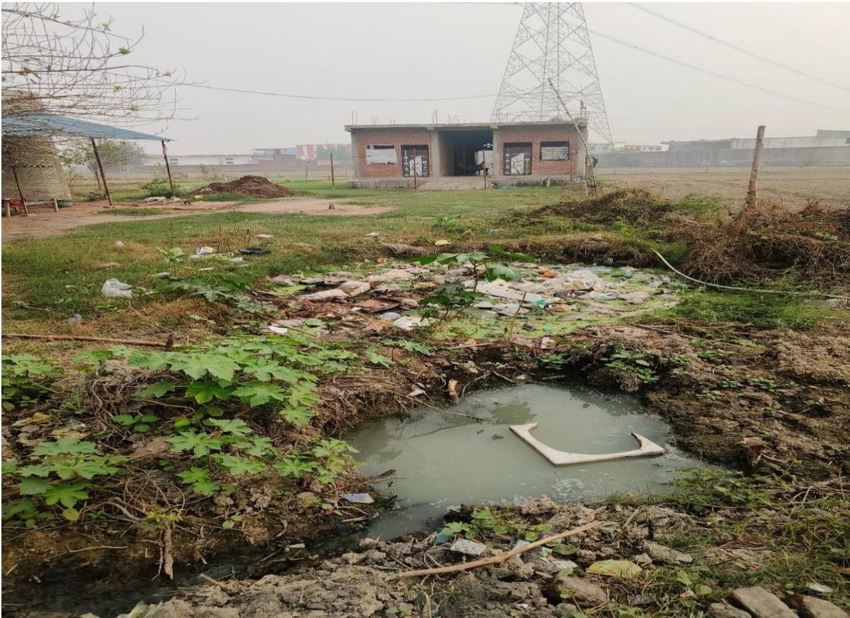
Image 32: waste water and solid waste being collected on vacant village land
