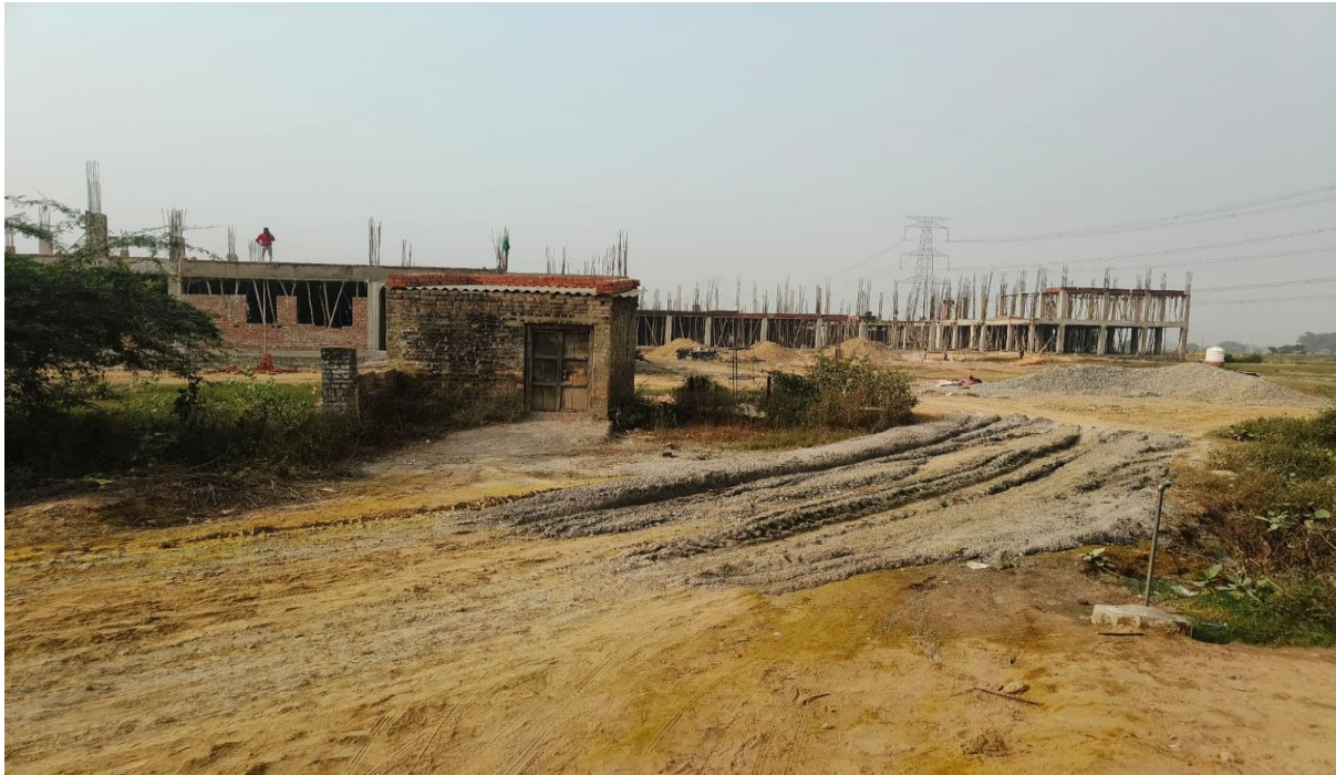
Image 54: construction site of educational institution near chromium dump
