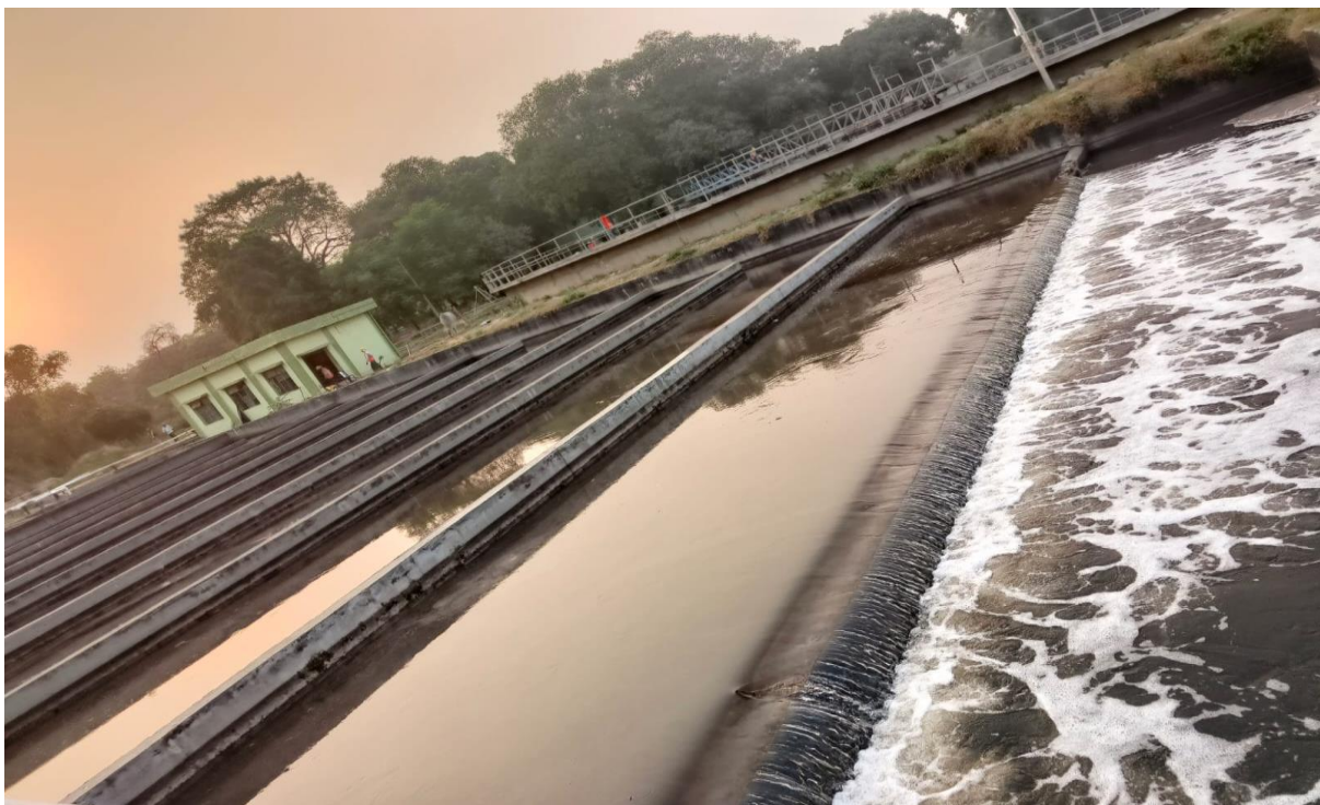
Image 16: outlet of 130 MLD STP (after chlorination)
