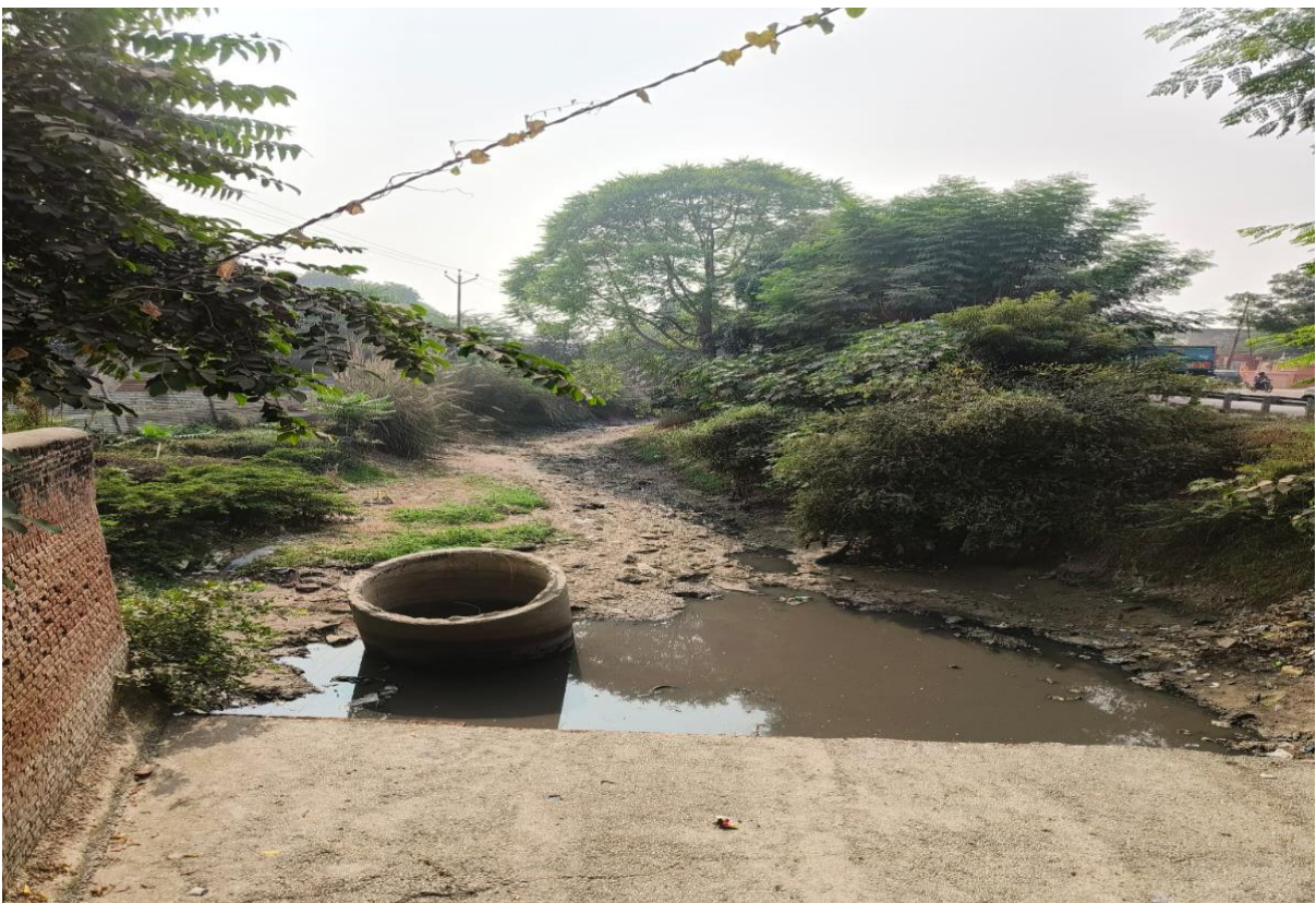
Image 11: discharge found in the COD drain post pumping station
