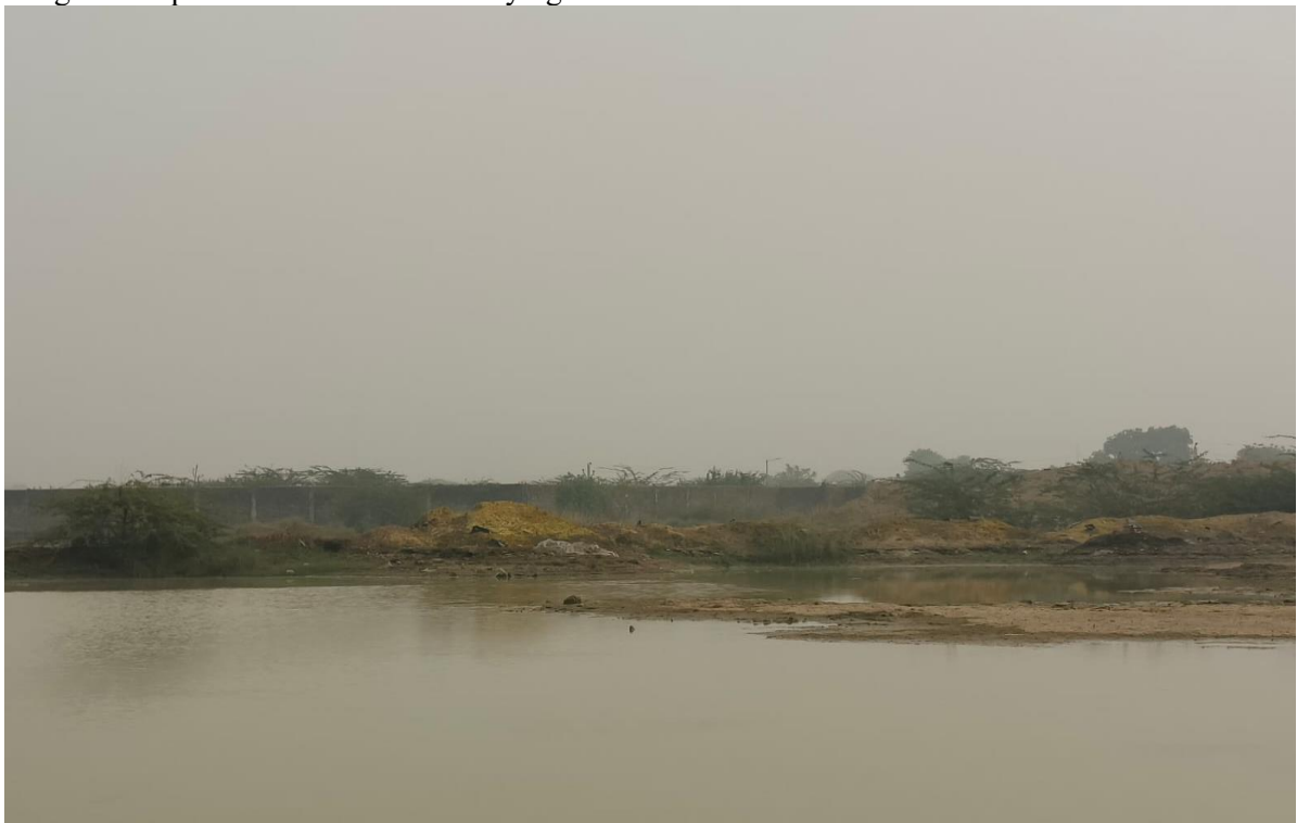
Image 23: Water has collected in the excavated site
