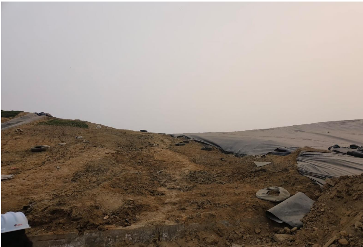
Image 40: M/s Bharat oil landfill site with treated waste (for ash they were using some other facility). This facility has an ETP for treating and disposing leachate and tyre wash.
