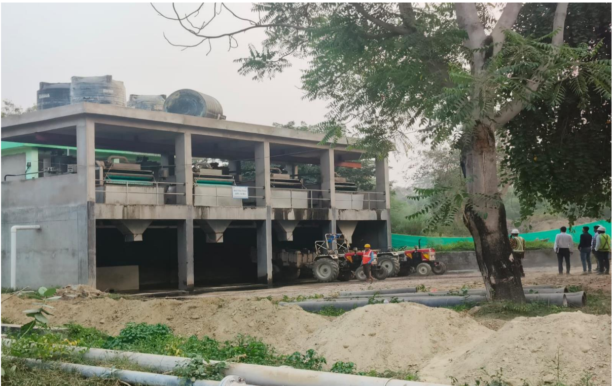
Image 18: sludge collected at the STP 130 MLD
