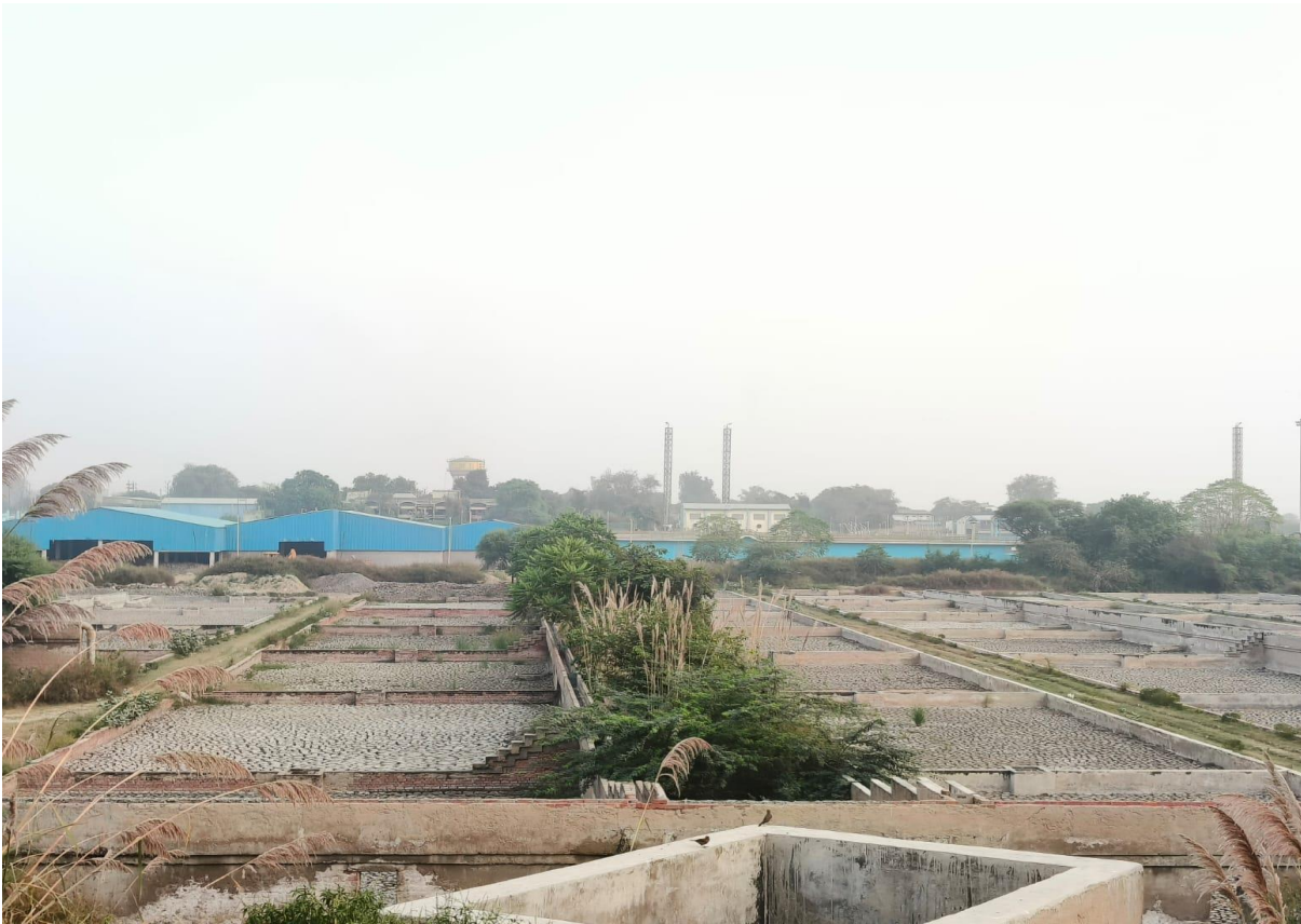
Image 19: dried sludge bed near the STP area
