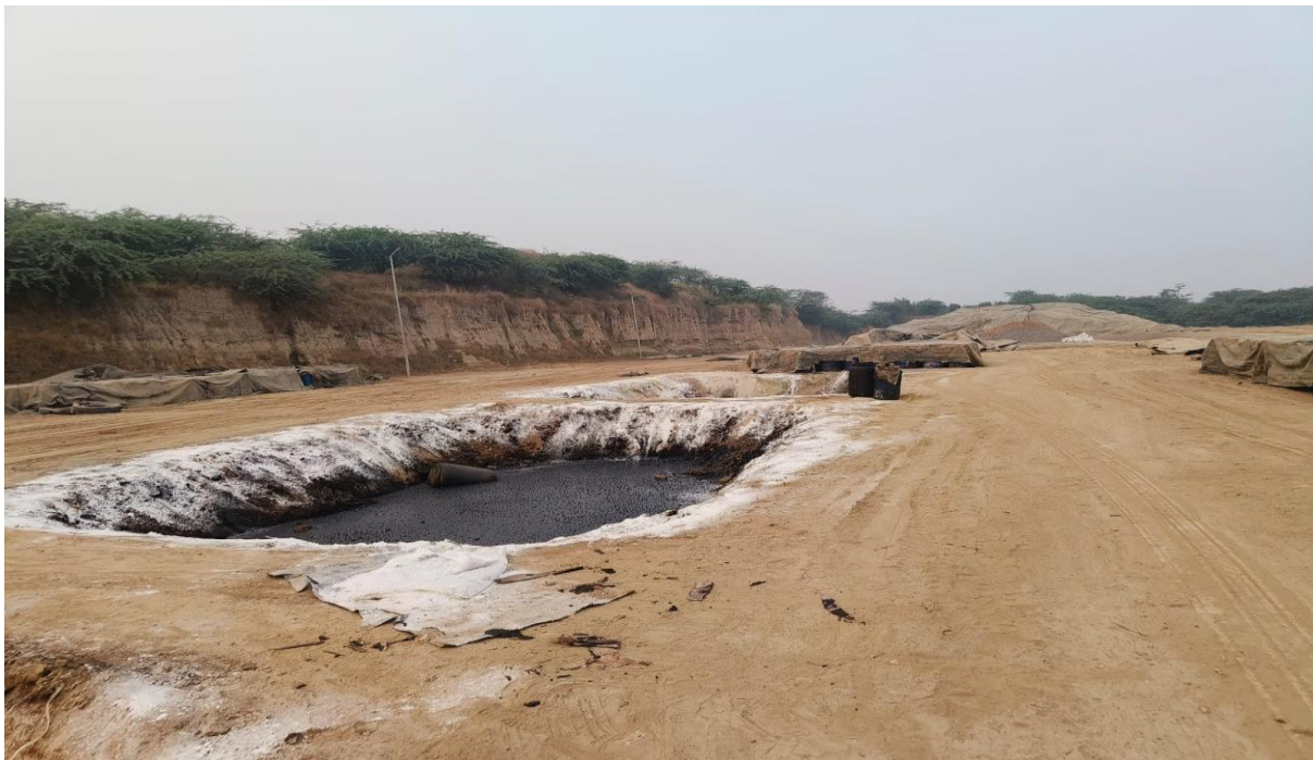
Image 38: huge ponds created to treat and stabilize Cr VI (with acids)
