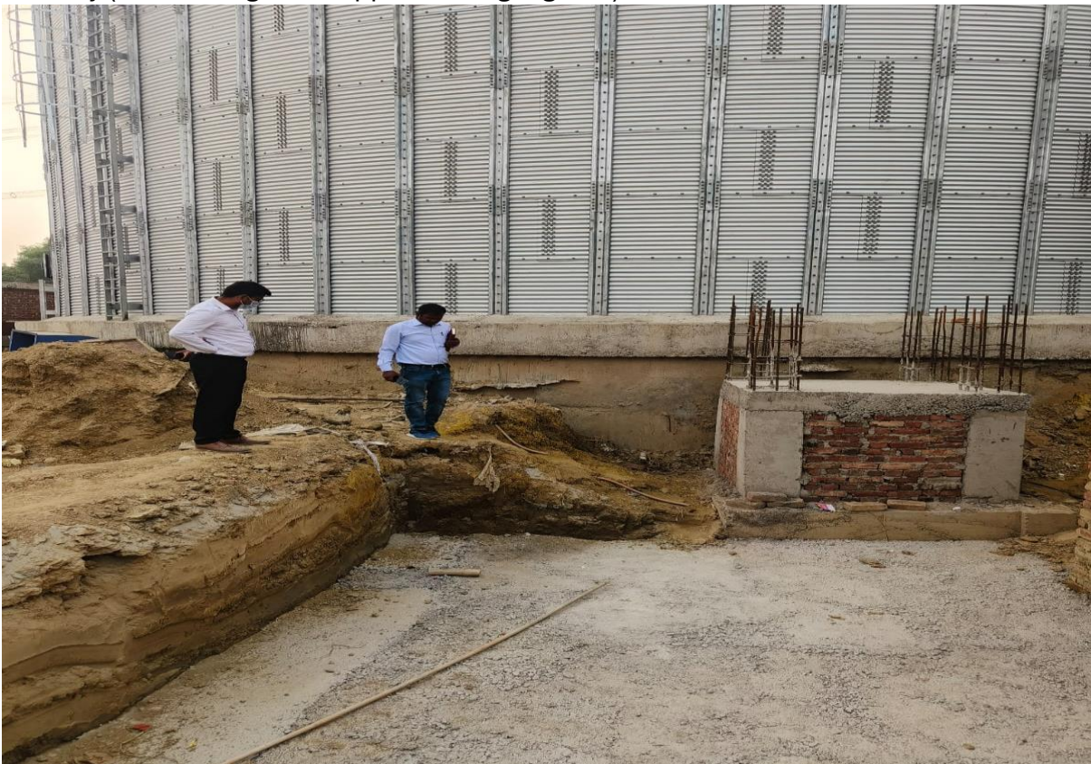
Image 57: the under construction flour factory (where the ground appeared bright green)
