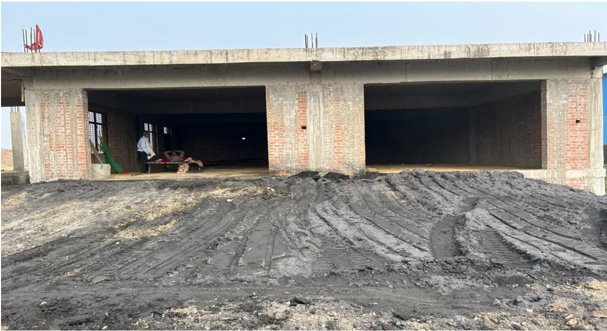
Image 35: Ash dumped and used for land filling
