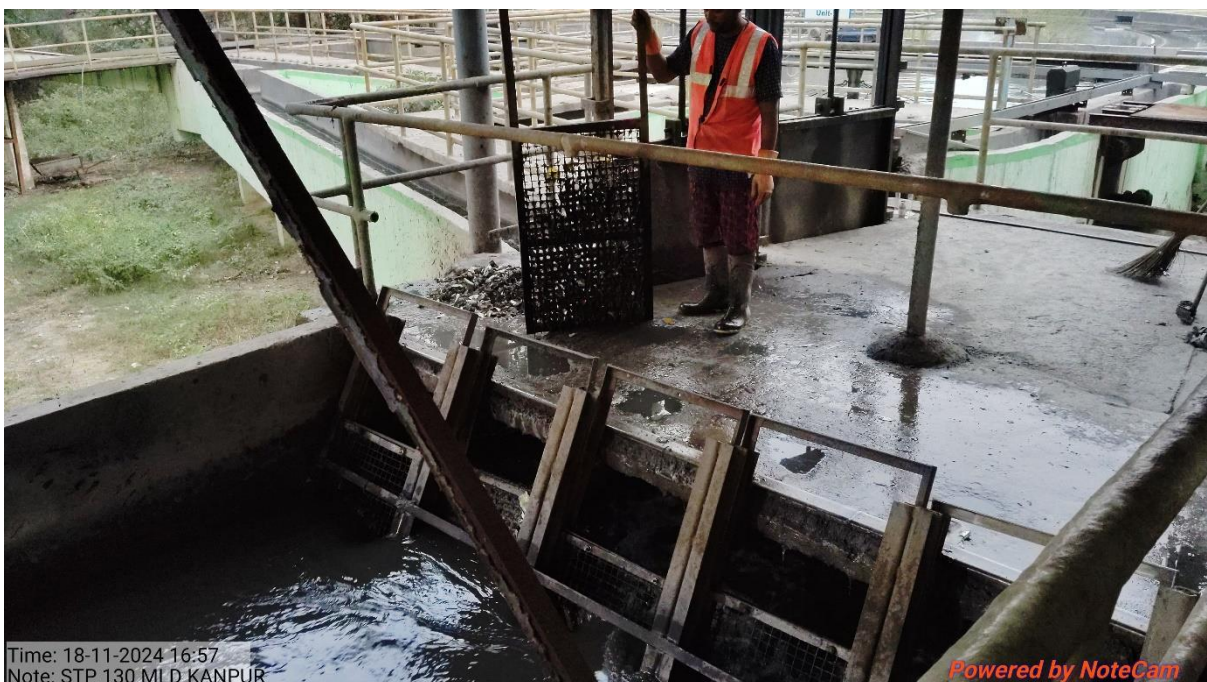
Image 14: inlet of Jajmau STP 130 MLD showing tannery waste
